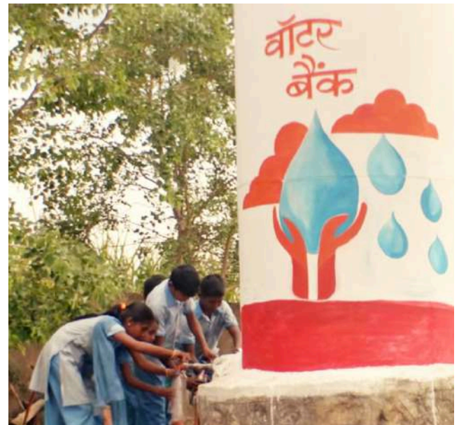
Rainwater harvesting project installation at a government school in Shivali village, Latur district, Maharashtra.
